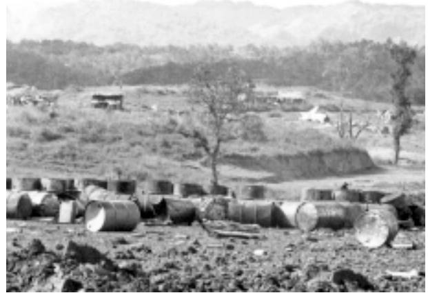
Destroyed fuel dump at Muong Suoi. All fuel had to be flown in in drums or large rubber bladders.
