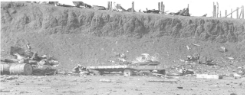
Bomb Damage at Muong Suoi. Note damaged "farm wagon" used to receive cargo from C-123Ks and C-130s.
