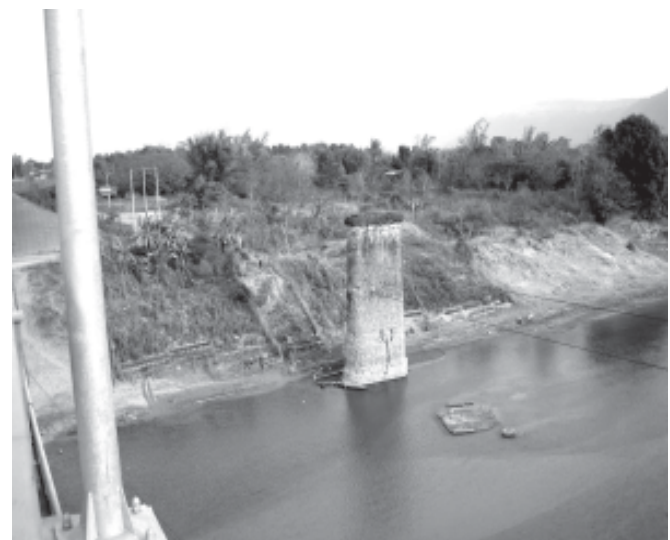
Original supports for the French steel girder bridge that used to carry Route 9 across the river at Tchepone, taken from the modern new concrete bridge that carries cars, trucks and buses from Vietnam across Laos to Thailand at Mukdahani.
