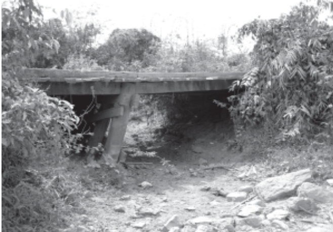
Typical wood bridge on the old Ho Chi Minh Trail. Many bombs were flung at these easily-built structures.
