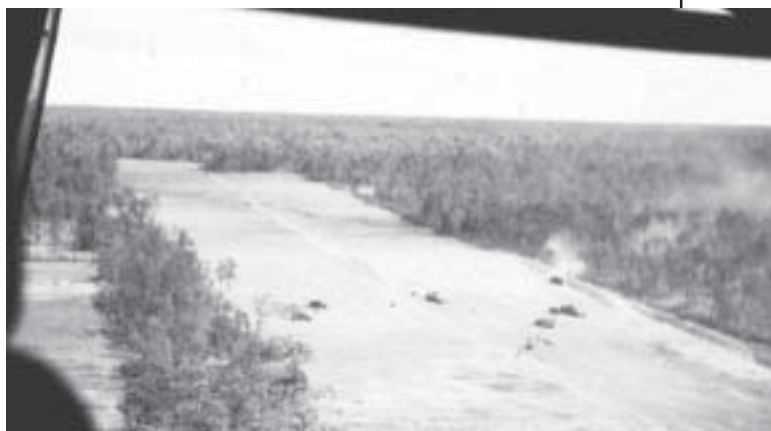
After the June 1963 opening ceremony, several C-130s landed and all but 35 Seabees boarded them to return to the states. Lt JG Fowler was OIC, stay-behind team. In November, the rains stopped and Seabees returned to NKP to finish the airfield.
